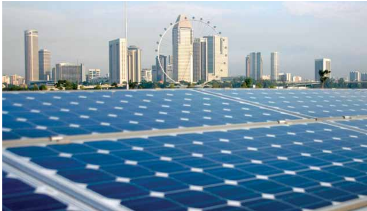
Solar panels on Marina Barrage building in Singapore.
