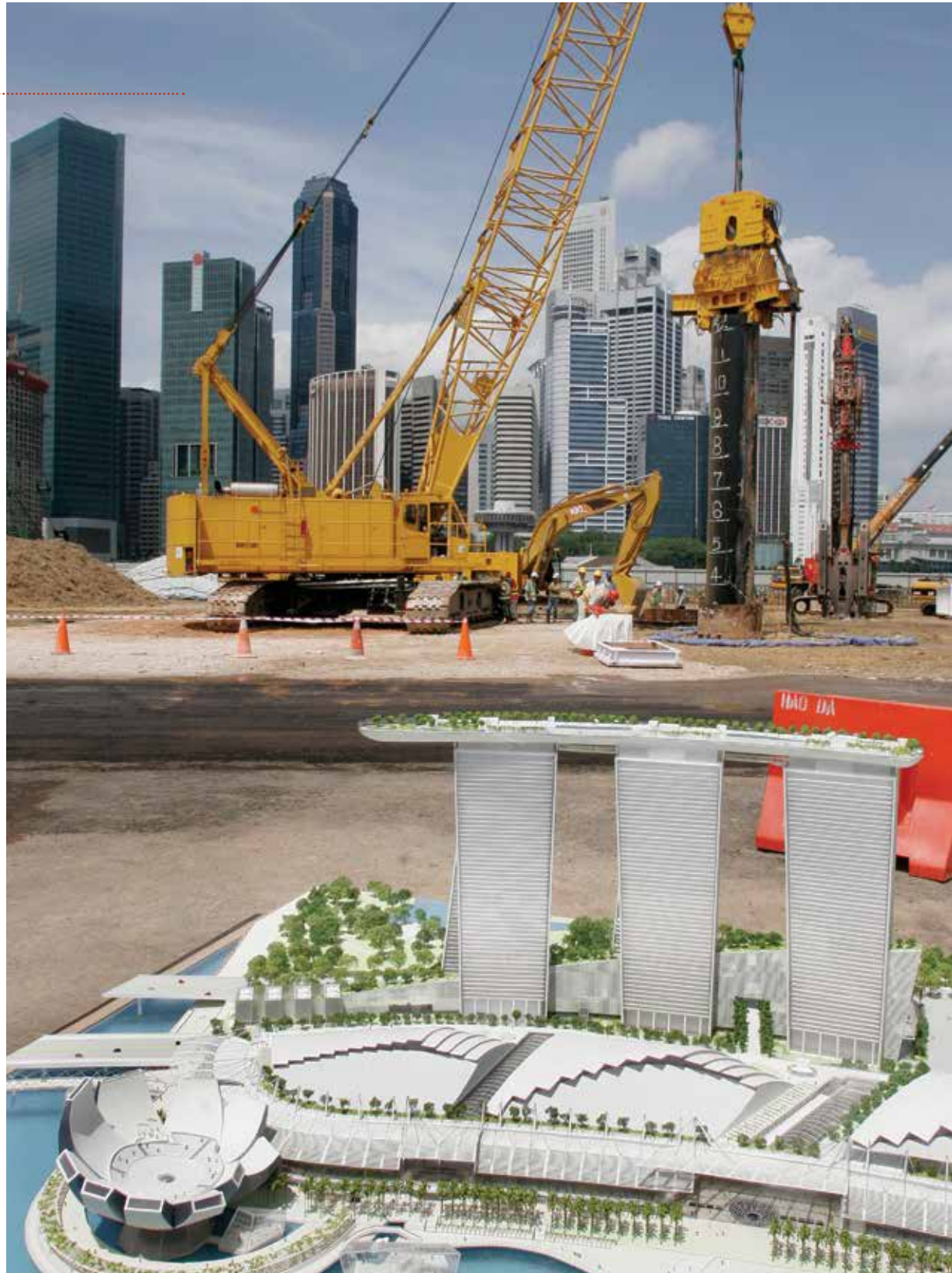
Work starts at a Singapore resort, with the city in background and a model of the Marina Bay Sands in foreground.
