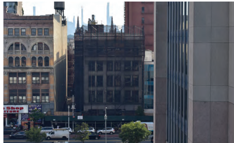
Construction at the Studio Museum in Harlem, September 2019
